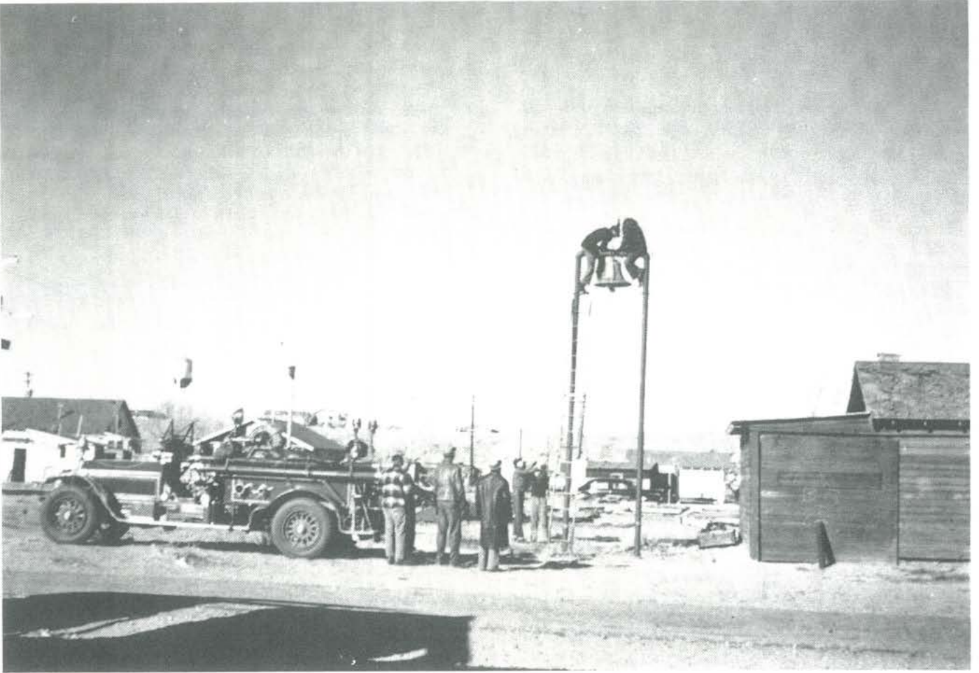
Work on the fire bell at the old hose cart building at Fourth and Wasatch, before construction of the fire hall. Courtesy Bert Harris.
