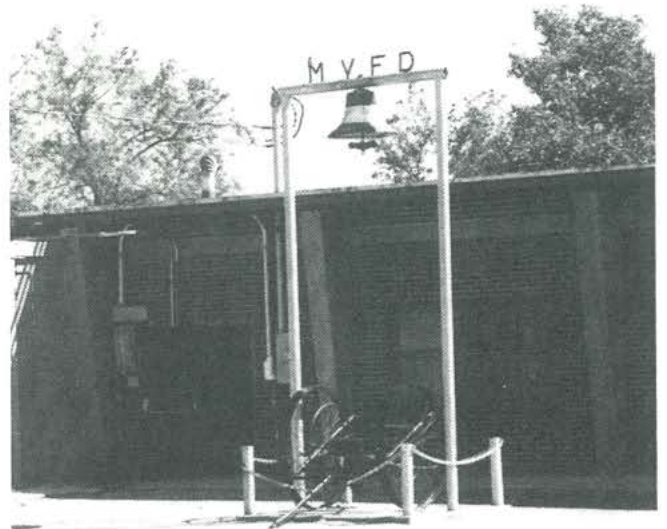
The Mills fire hall. Note the hose cart and fire bell. The hose cart was pulled behind a fireman's car (whoever got to the fire hall first) to the fire, where the hose was hooked to a hydrant.
