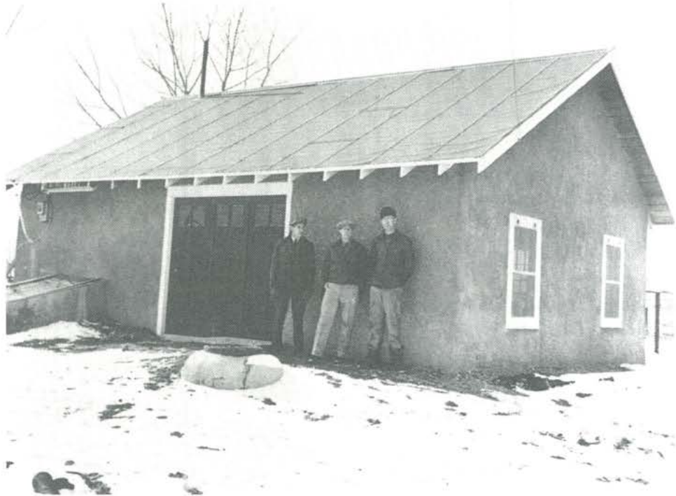
O. V. Patterson, Fred Steinle, and Ted Stamper at the Mills pumphouse.
