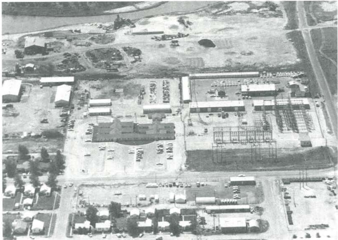
Aerial View of the Bureau Of Reclamation site, looking south, 1969. Note the Boatright-Smith site and the North Platte River to the south. The large office building in the center has been replaced by an office building located to the bottom of the picture. A new operations center has been built also. Photo by B. F. Cronin. Courtesy U.S. Bureau Of Reclamation.
