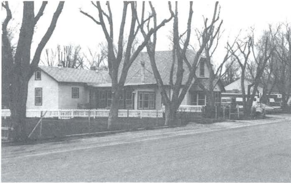
The George Sword house at Second and Benton, earlier the home and store of George Boyle, first mayor of Mills. Well taken care of and also representative of the early days.
