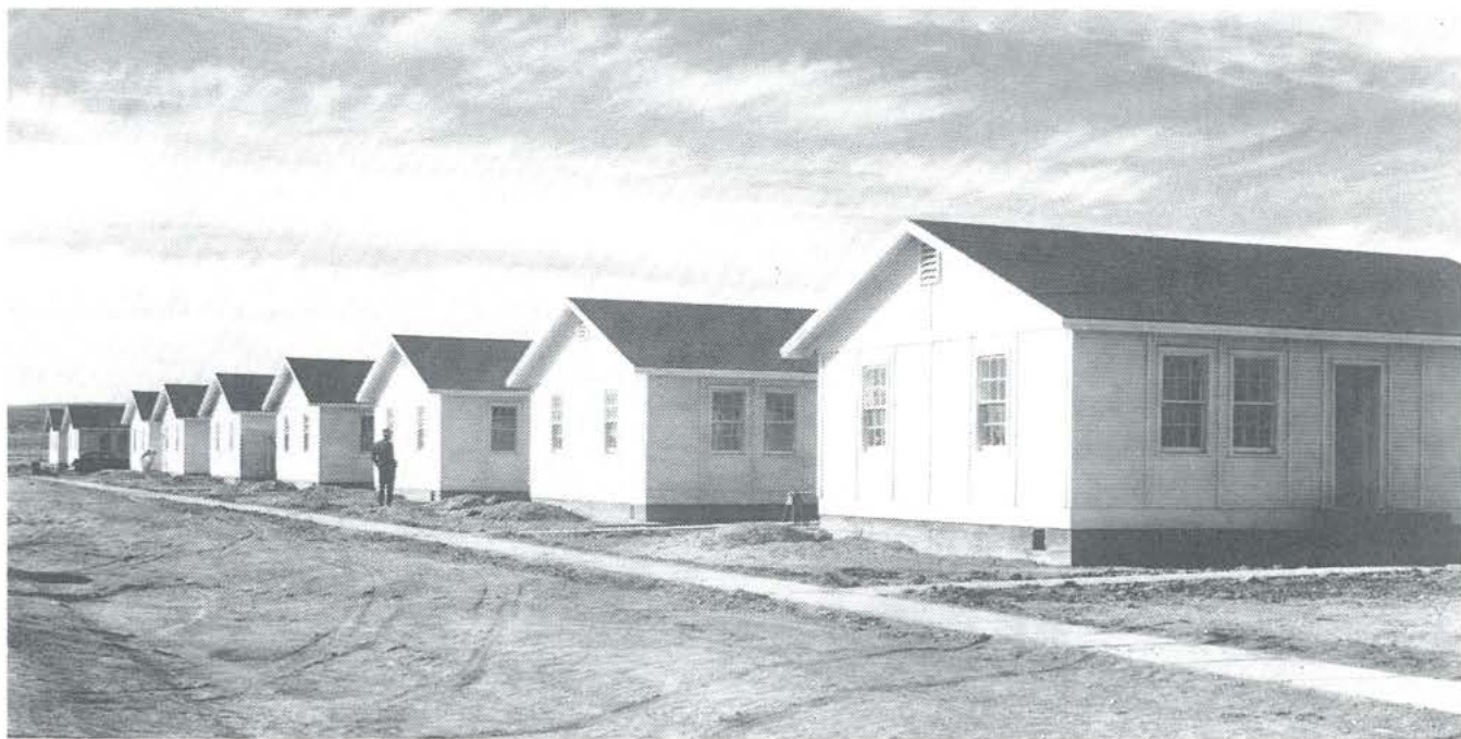
Bureau Of Reclamation housing being constructed in 1947, when the Bureau was the Mills Camp of the Kortess Unit. These homes, built as two bedroom, prefabricated units, were eventually sold to the public and are still being put to good use today. Photo by L. E. Bowman. Courtesy U.S. Bureau Of Reclamation.
