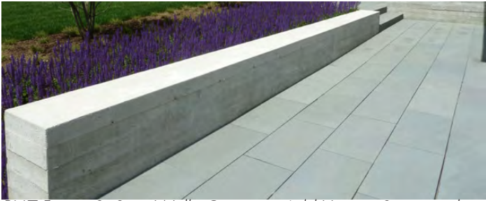
PH7 Figure 3: Seat Wall - Option to Add Veneer Stone and Cap.
