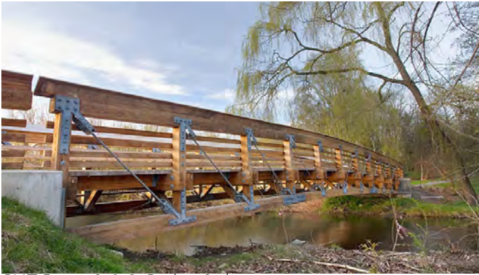
PH7 Figure 1 & 2: Bridge Style
